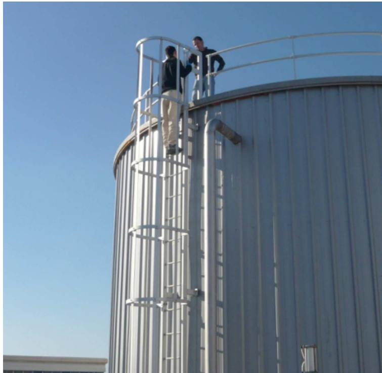
(a) A single-reactor design. An example of this design is found in Spain.
