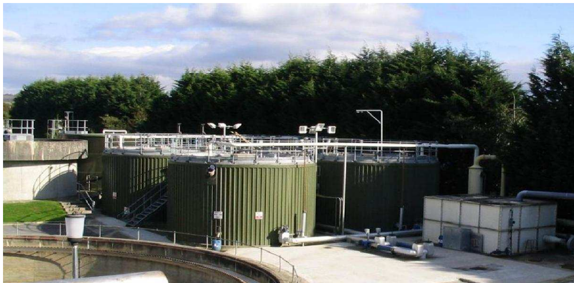
(b) A two-reactor design. Semi continuous or continuous treatment requires multiple reactors to achieve pasteurization. An example of this design is found in Killarney, Ireland.
